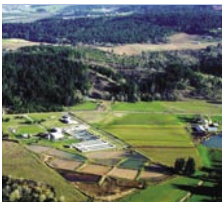
Current JWC Treatment Plant
