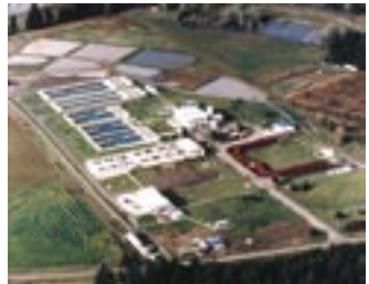
JWC Treatment Plant
