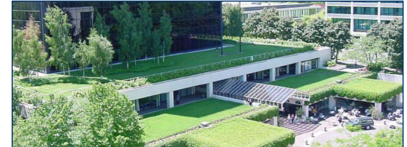
Bioretention Areas Buckman Heights , Courtesy: City of Portland
