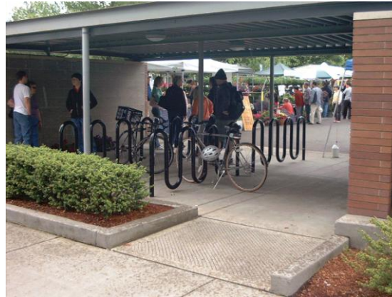
Covered long-term parking keeps bicycles and riders protected from the weather. (Ribbon rack design is not recommended.)
