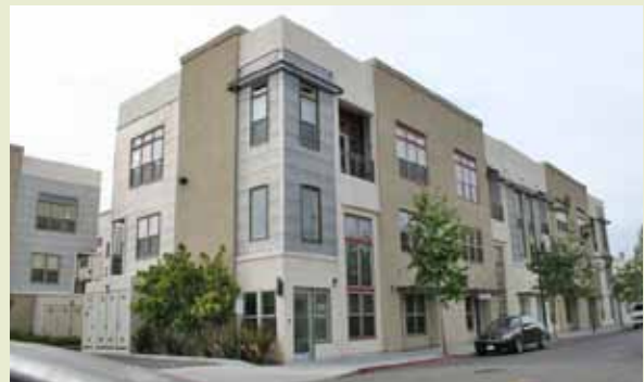
Three-story, mixed-use development in Portland.
