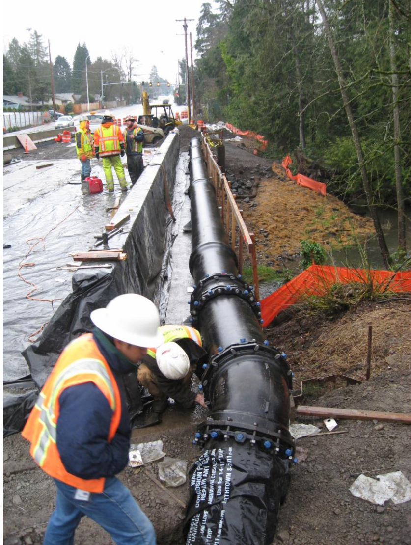
Water Extra Capacity Project
